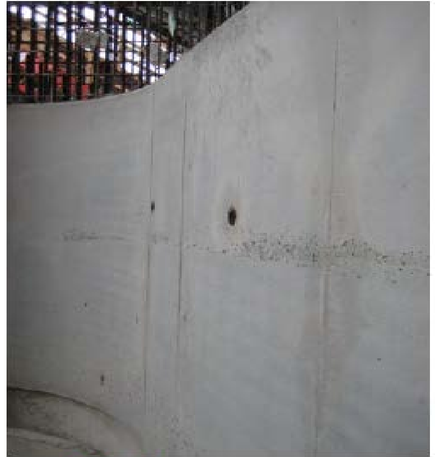
Left: Concrete finish quality issues at 70 per cent GGBS replacement Right: Approved finish surface, achieved without any rework at 40 per cent GGBS replacement and 76 per cent coarse aggregate replacement
