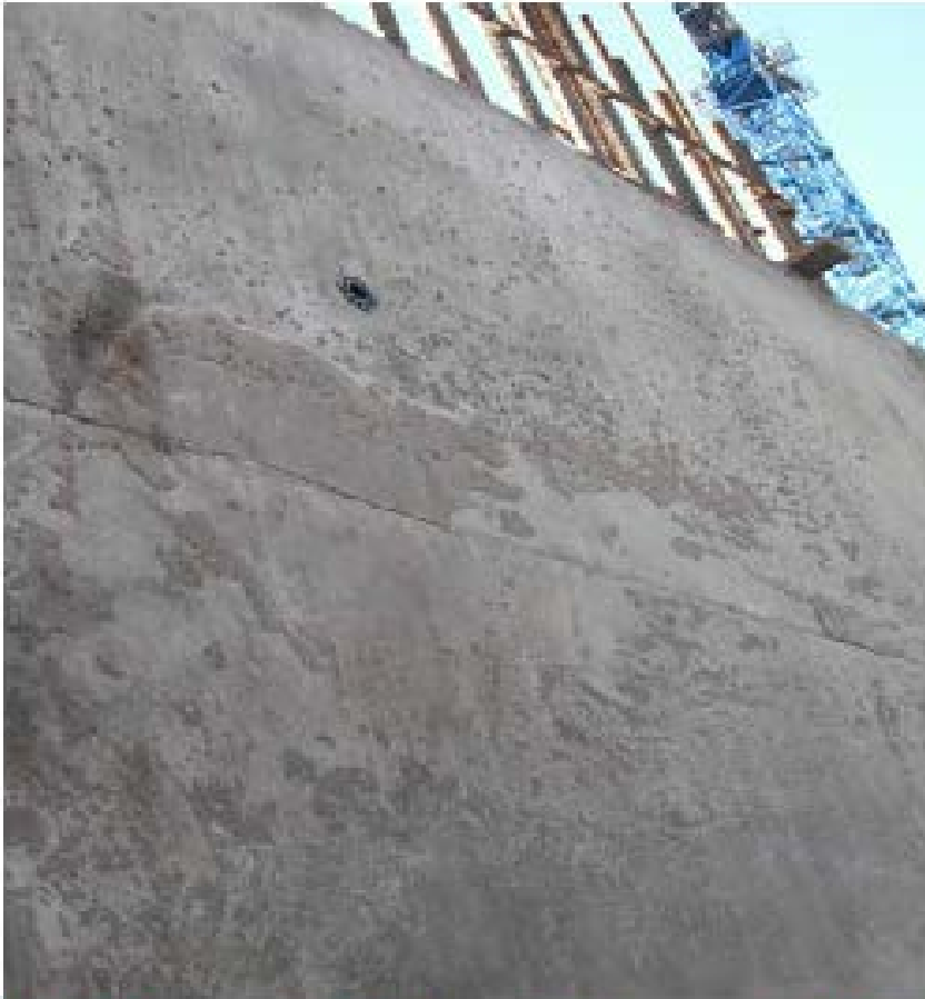
Left: Concrete finish quality issues at 70 per cent GGBS replacement Right: Approved finish surface, achieved without any rework at 40 per cent GGBS replacement and 76 per cent coarse aggregate replacement
